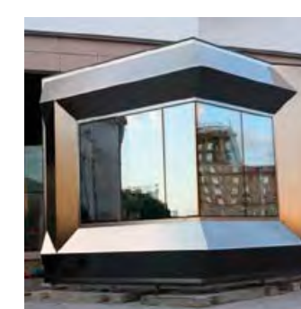
Kulneva, Moscow The 2,000 mm-wide basic material was dyed half in champagne, half in black using a multi-spectral process. It was then edged and relief-milled in one piece in order to obtain as low an edge radius as possible.
