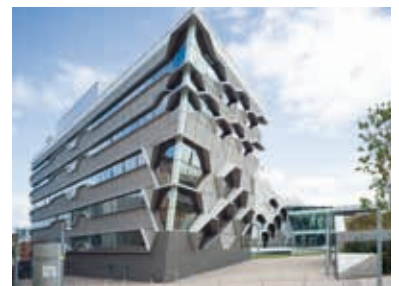
CUEB_M171 view west 4
