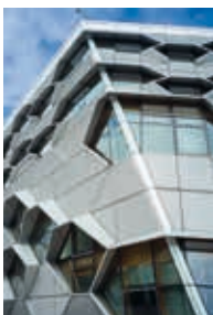
CUEB_M159 view southeast 5
