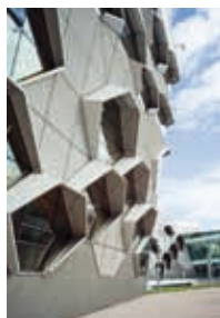
CUEB_M168 view west 3
