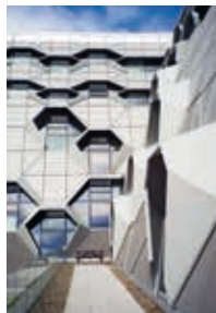
CUEB_M150 view southeast 4
