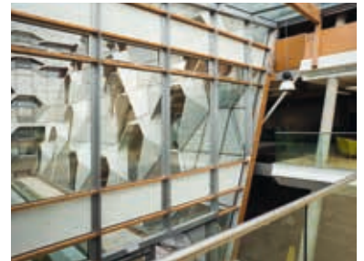
CUEB_M141 view foyer south
