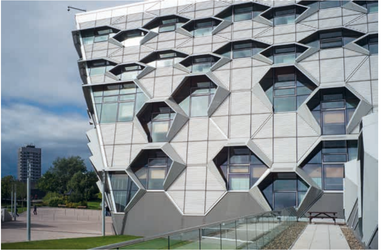
CUEB_M152 View View Southeast 1
