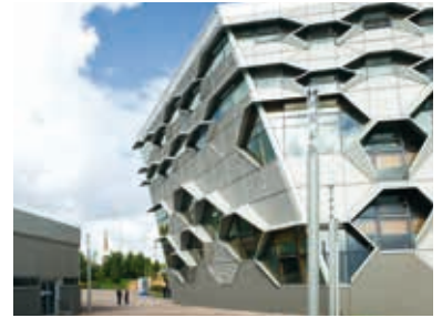
CUEB_M106 view southeast 3
